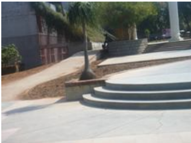
Ramp in Main Building
