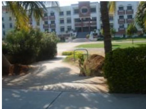
Ramp in MNS Block
